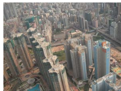
New highrise residential developments in West Kowloon development - slender tall blocks will have less obstruction to air flows, but spacing and layout of the blocks should take account of the direction of the prevailing wind.
